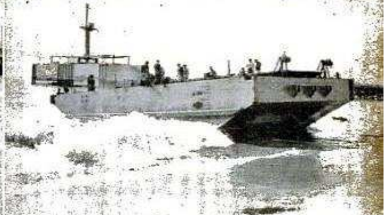
Barge uses propeller (which can be set at various angles) as far up the shore as possible before starting to walk. Outbound, it reverses process and walks as far as it can.
